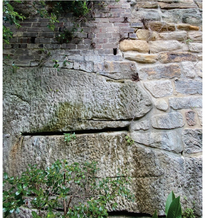
Retaining wall materials
