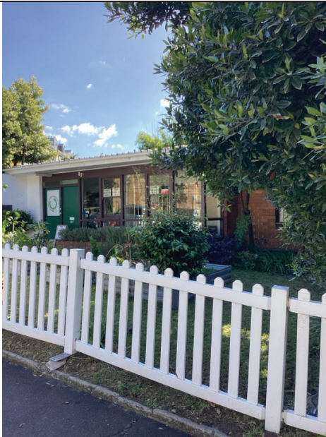
Figure 14 Existing fencing on site
